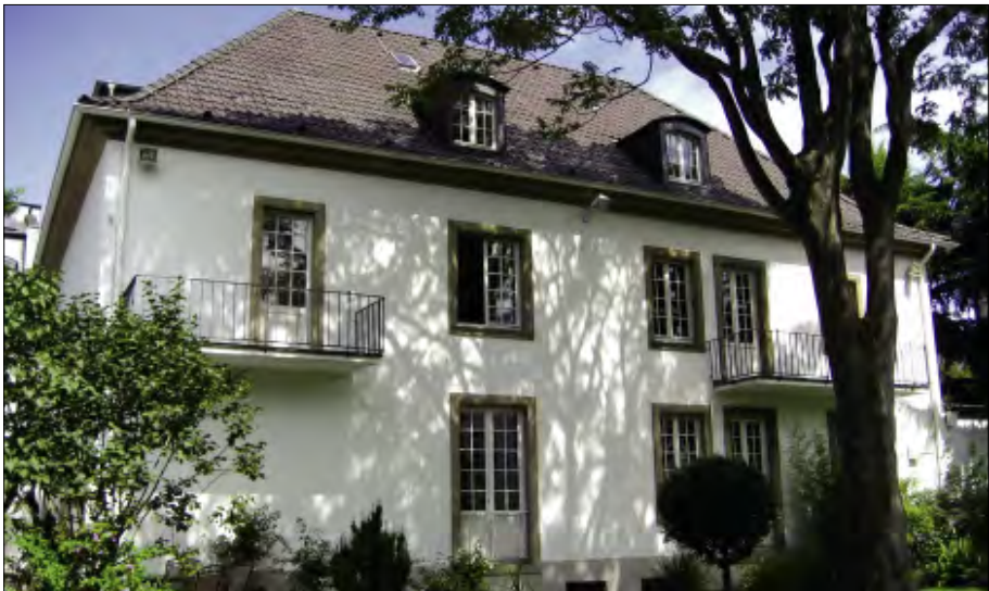
Bundeskartellamt, building III
